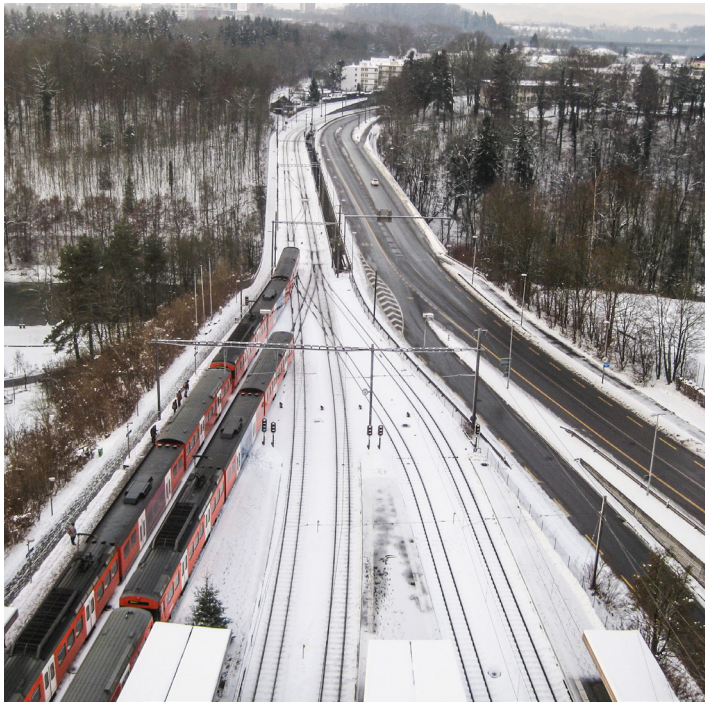
Siemens' ZSL 90 train protection from the 1990s has earned a reprieve on Berne-Solothurn Regional Railway (RBS), but ZBMS remains a long-term option. Markus Enzler captured Worblaufen station, where three routes converge, on 14 December 2012.
