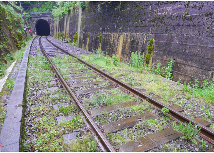
The 2.1 km Rosshäusern Tunnel will replace an existing line segment, 300 m longer, whose 116-year-old infrastructure needs major repairs.
