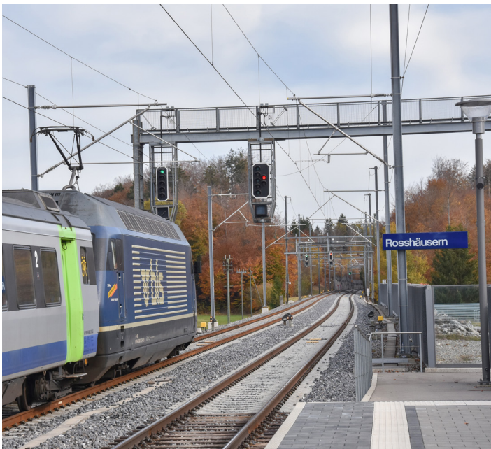
BLS rebuilt Rosshäusern station but retained its Siemens Domino 67 interlocking and the signals for the since-lifted points of a third track that served industries here. Eastbound drivers thus see three sets of signals within 530 metres.
