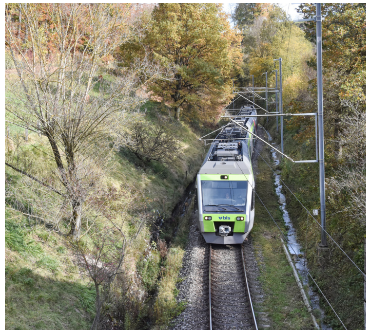
Trains on the existing line run through a deep and sinuous cut that they share with the Flüelebach, a troublesome stream.
