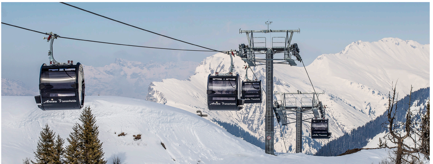
A gondola ropeway in the Lenzenheide ski region in eastern Switzerland in March 2016. The gondolas detach from the moving cable momentarily while people board and alight. Photo BMF.
