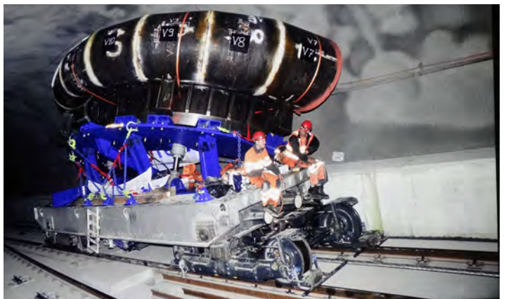
A film showed that the inclined railway brought some large components in pieces. The 40-tonne wagons run at 6 m per second empty, but at only 0.5 m per second when carrying their maximum load of 215 tonnes. Photo Markus Grämiger.
