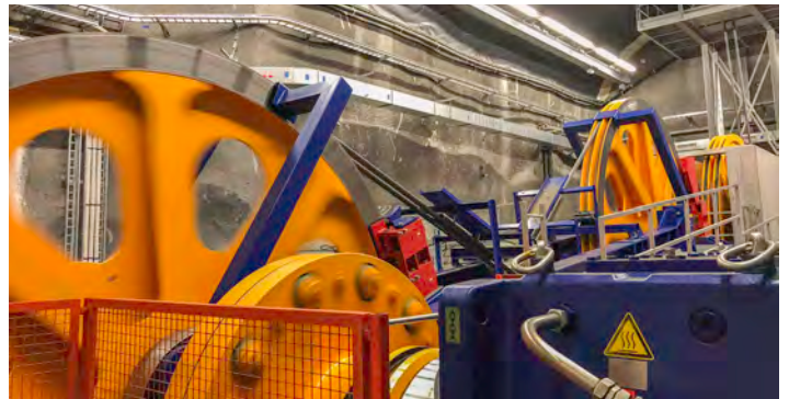
Two motors rated at 870 kW each power the inclined railway’s cable. Photo Peter Hefti.
