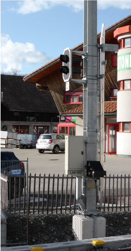
Left: A line signal and shunting signal and the connection box for both.
