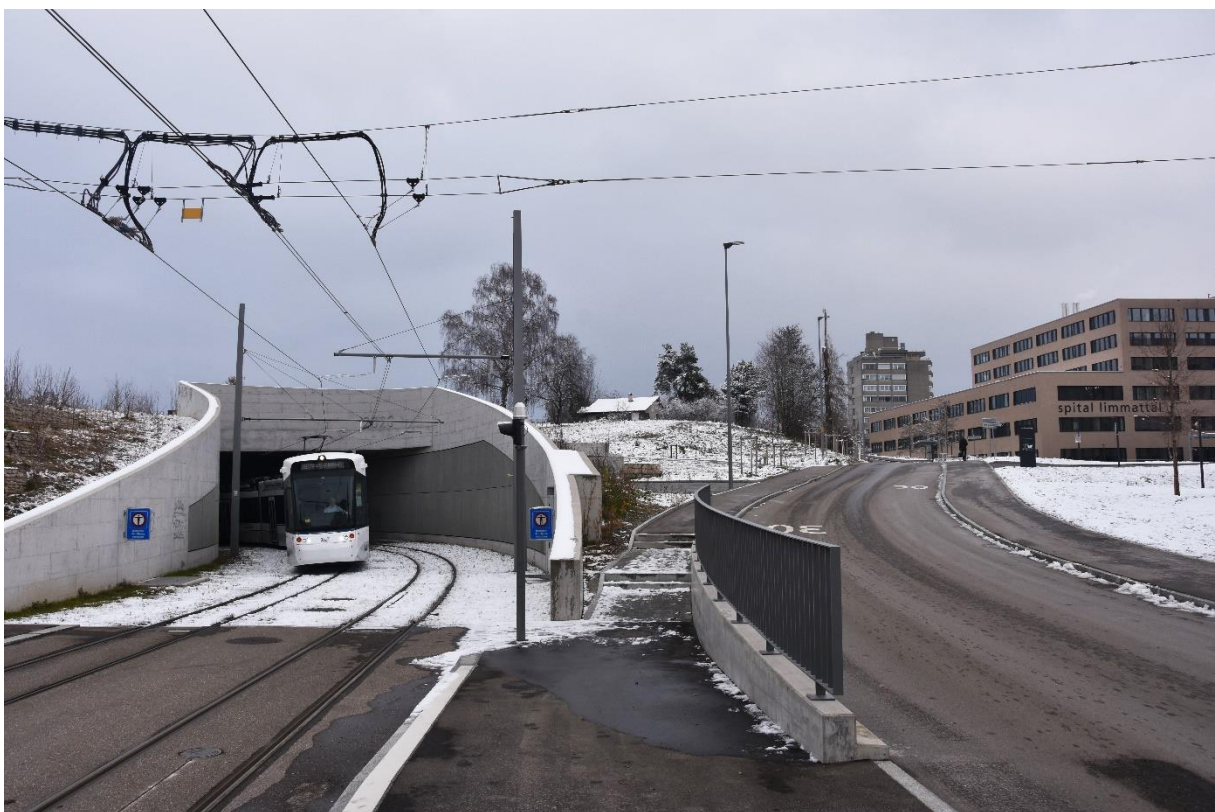
A westbound LimmattalBahn train emerges on 12 December 2022 from the 245-metre Färberhüsli Tunnel to serve Schlieren's Limmattal Valley Hospital, whose new building opened in 2018. Photo © George Raymond
