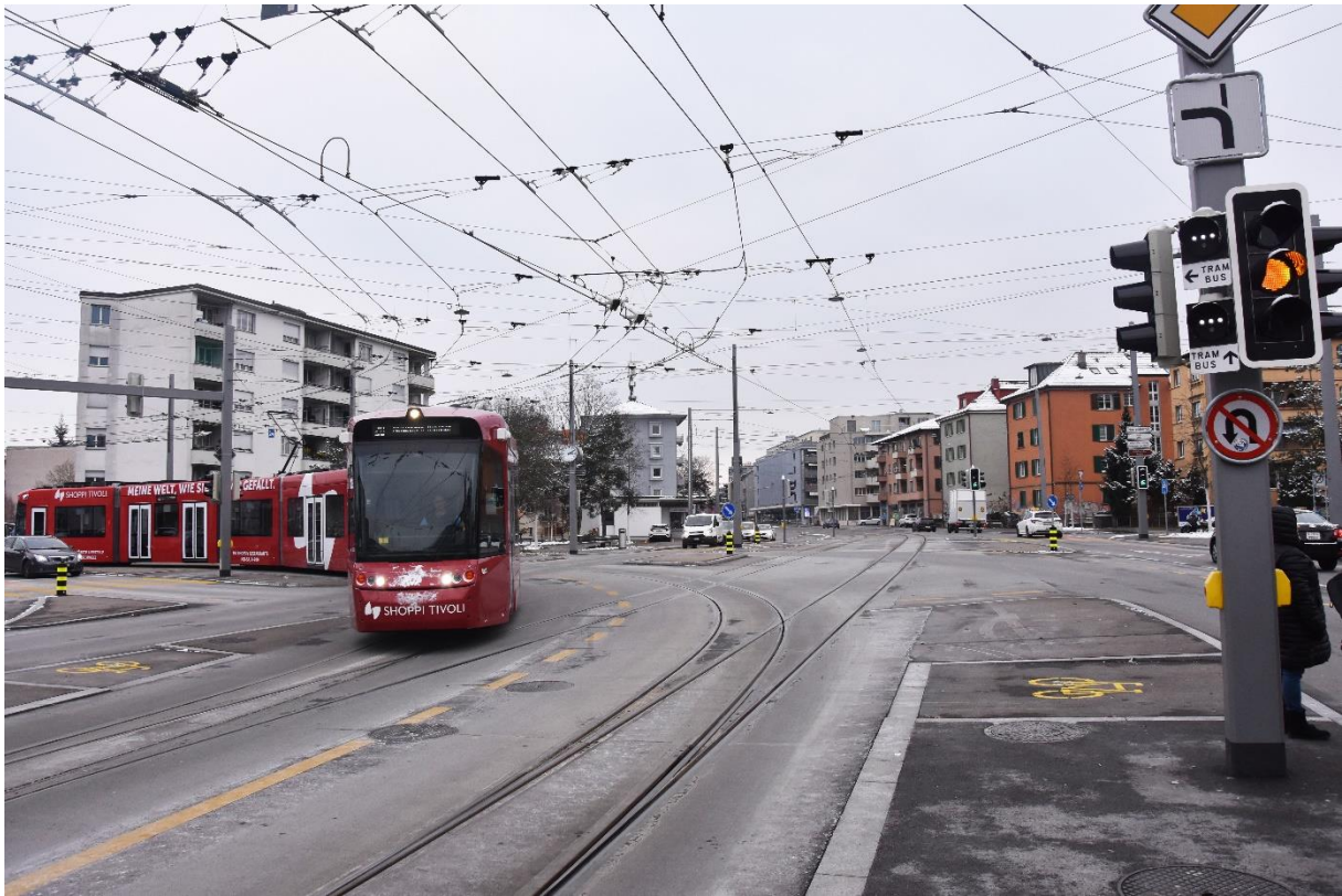
Proceeding west from Altstetten, LTB's tracks merge with those of Zurich tram 2 at Farbhof. A westbound LTB train swings its seven sections on 12 December 2022 into Farbhof station, which it also shares with trolleybuses, as the catenary shows. Photo © George Raymond
