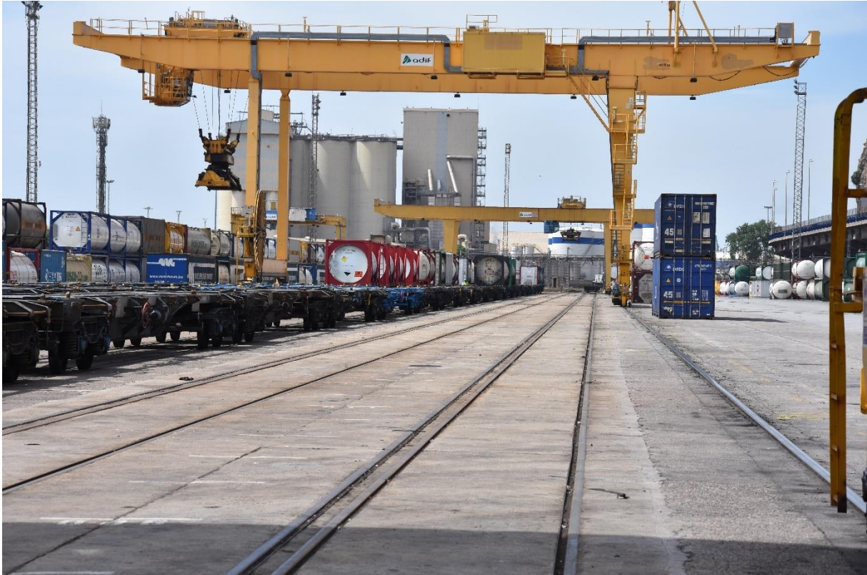
Three-rail track to handle both standard (1435 mm) and Iberian (1668 mm) gauge wagons. Morot terminal, Barcelona. 9 June 2016. Photo George Raymond.
