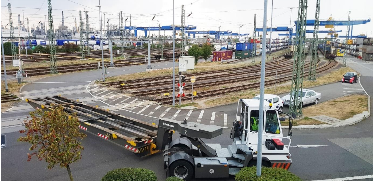
BASF's combined-transport terminal in Ludwigshafen, Germany. The Rhine is nearby. 6 September 2018. Photo George Raymond.
